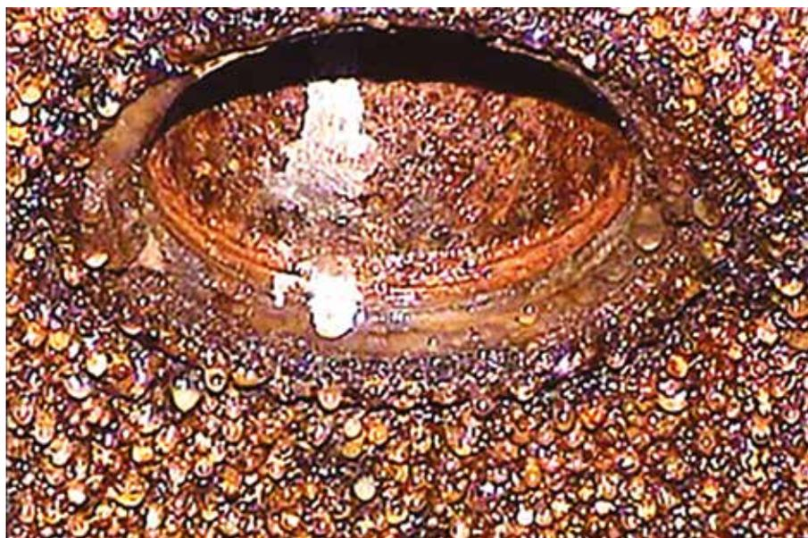
**Condensation droplets and corrosion near the bung at the top of an Underground Storage Tank, captured on video using Tanknology's TankCam Video Inspection System.**
