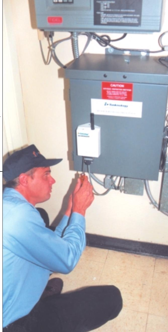
Corrosion technician finalizes installation of cathodic protection system remote monitoring unit.
